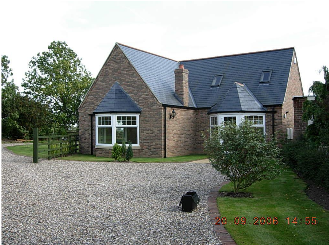
Appendix reference 3. Photograph showing existing driveway and associated turning.
