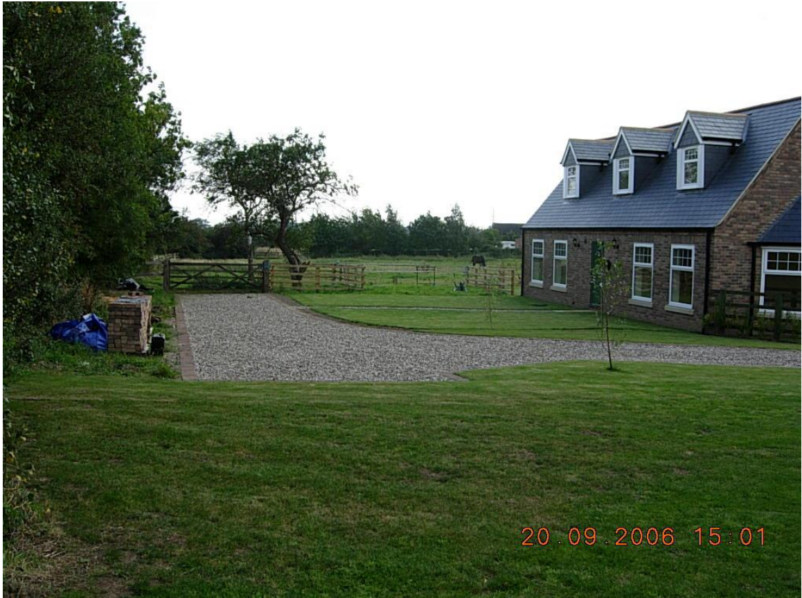
Appendix reference 8. Photograph showing works undertaken to agricultural land, including access track and its current character and appearance.
